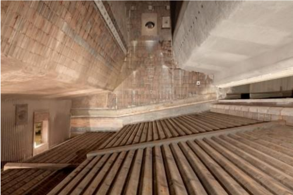
Figure 12. Reststoffen Energie Centrale, Harlingen, The Netherlands
