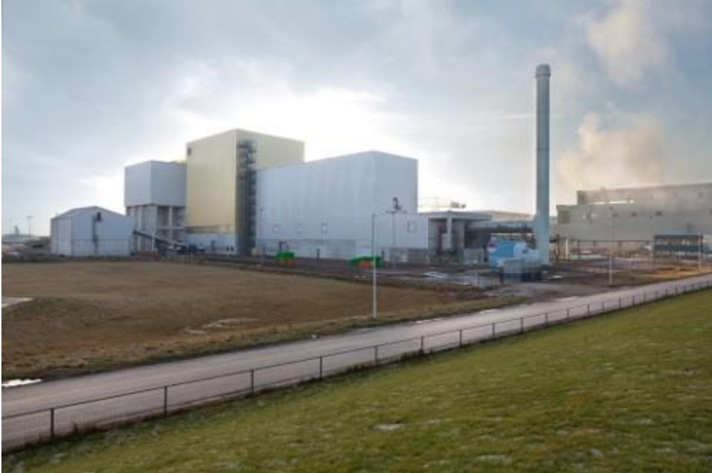
Figure 11. Reststoffen Energie Centrale, Harlingen, The Netherlands
